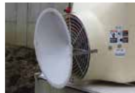
Wind deflector cones can be easily adapted to new or existing fans to improve the efficiency and performance of the total ventilation system.
