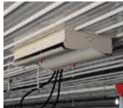
ACI-4000P2 ACTUATED CEILING INLET
