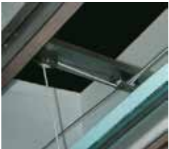
Actuated ceiling inlets include factory installed pulleys
