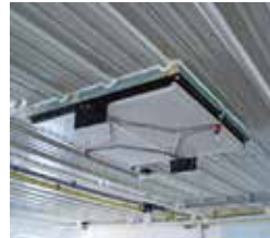
ACI-2700 ACTUATED CEILING INLET
