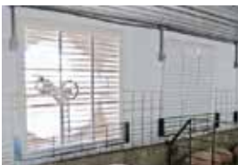
Standard white PVC* shutter with plastic rod hinges
