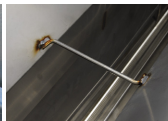
WELDED CENTER BRACING
